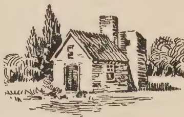
FIG. 4. TOWN SCHOOL AT DEDHAM, MASSACHUSETTS, BUILT IN 1648
