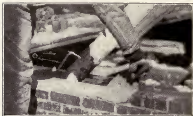
Fig. 28. — Throwing mortar on interior face tier.
