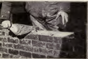
Fig. 26. — Buttering the end of the laid brick on the exterior face tier.
