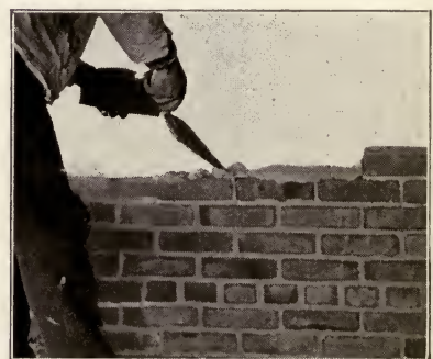
Fig. 33. — Handling mortar for two brick at one time on interior face tier.
