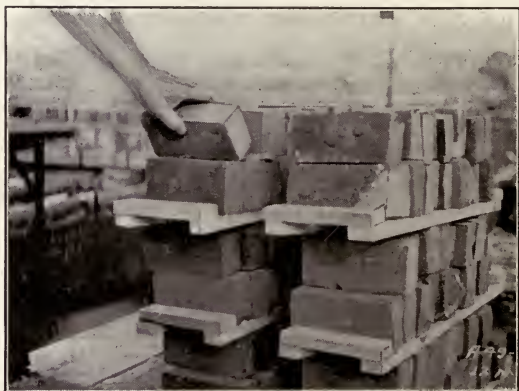
Fig. 5. — Wrong way to pick up brick from upper tier on the packet.
