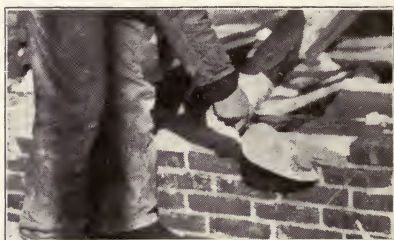
Fig. 30. — Cutting off mortar before brick is laid.
