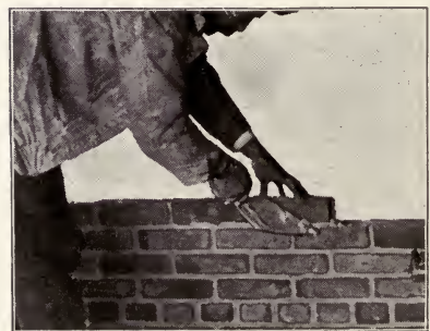
Fig. 32. — Cutting off mortar after brick is laid on interior face tier (here working left to right).
