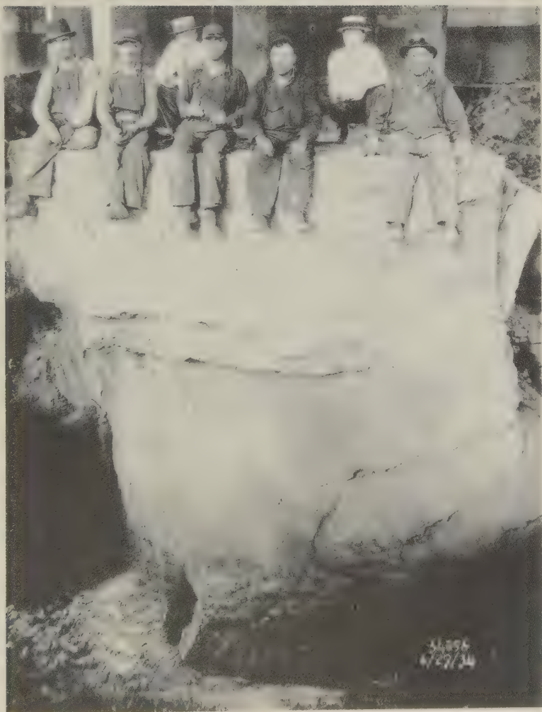
Blast furnace laborers sitting on an excavated concrete foundation pier during repairs at the blast furnaces, 1934.
