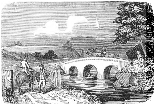
THE STONE BRIDGE AND TOLL-GATE.
